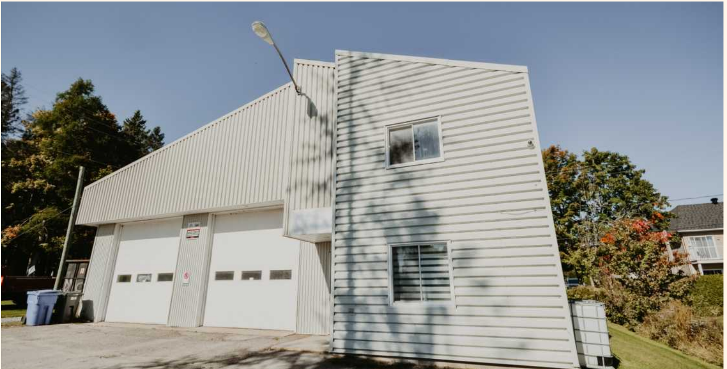
GARAGE MUNICIPAL (730, RUE OMER-BOUCHER)
